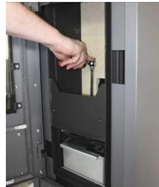
Fig. 77: unscrewing burner pot
