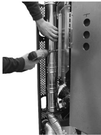
Fig. 63 - Pipe fastening
