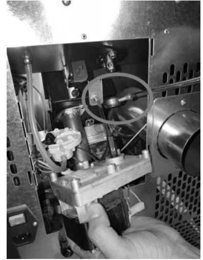
Fig. 71 - Gear motor removal
