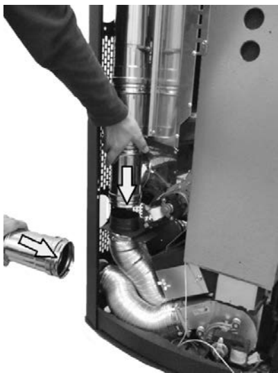
Fig. 62 - Pipe positioning for ducting
