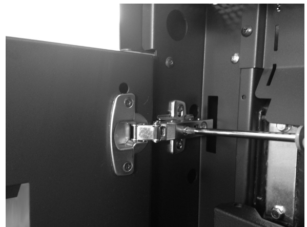
Fig. 44 - Door adjustment
