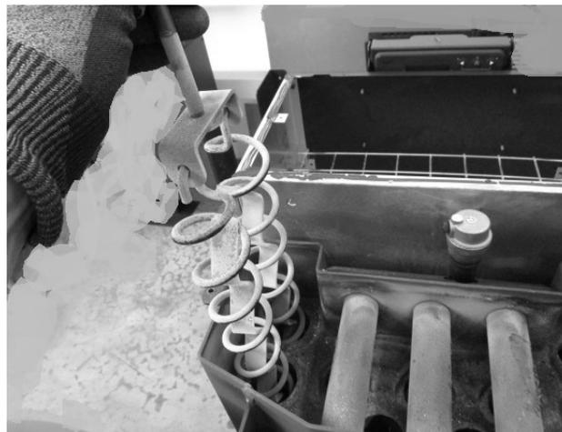
**Fig. 94 - Replacing turbulators if necessary**
