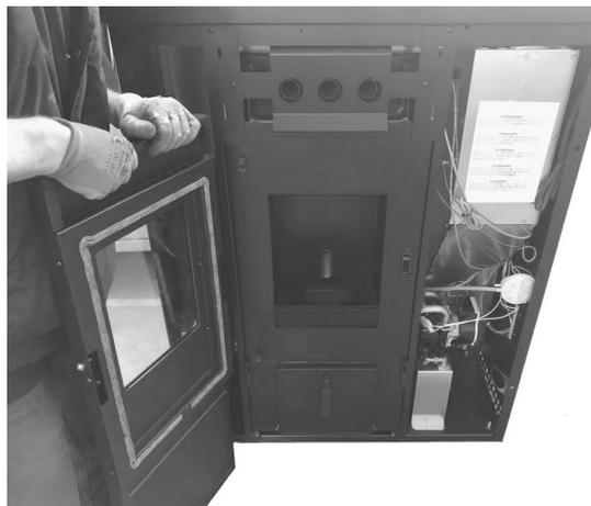
Fig. 20 - Remove the hinge
