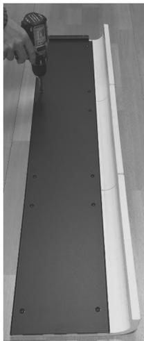
**Fig. 34 - Fitting the maiolica panels**
