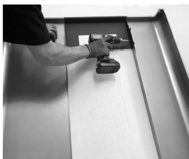
**Fig. 38 - Secure the strut**
