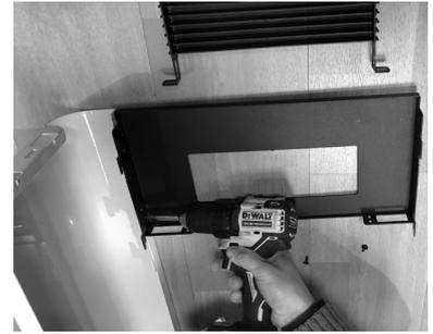
**Fig. 29 - Secure the panel to the support**
