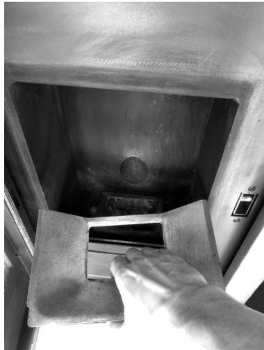
**Fig. 82 - Vacuum out the ash**
