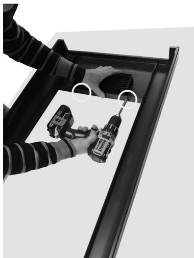
**Fig. 22 - Secure the grate**
