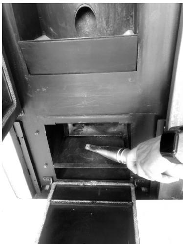
**Fig. 84 - Vacuum out the ash**
