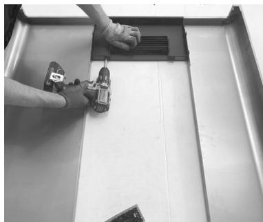
**Fig. 39 - Secure the grate**
