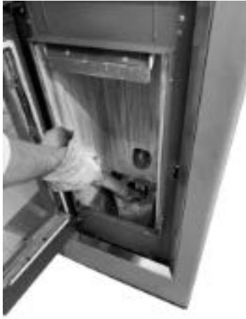
Fig. 35 - Burning pot box cleaning
